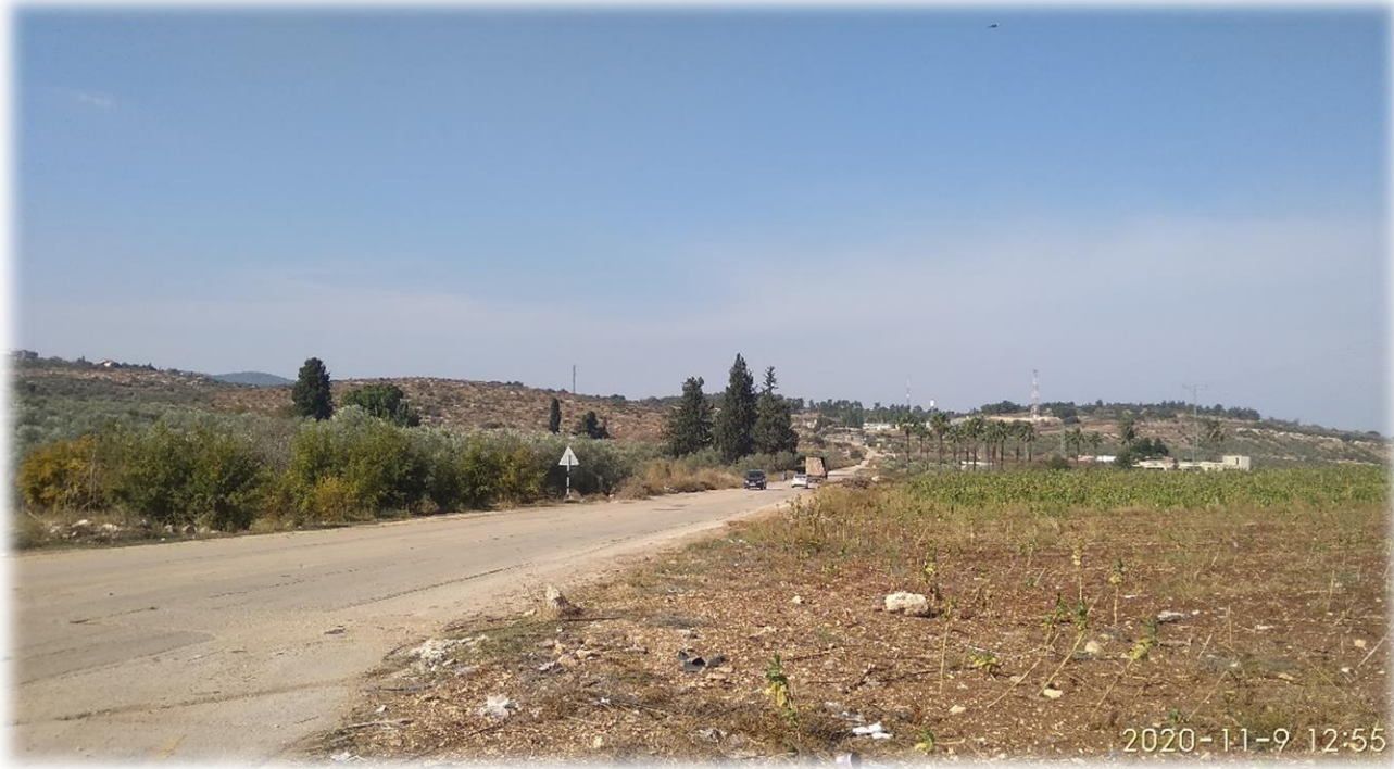
Salem Connection Point
