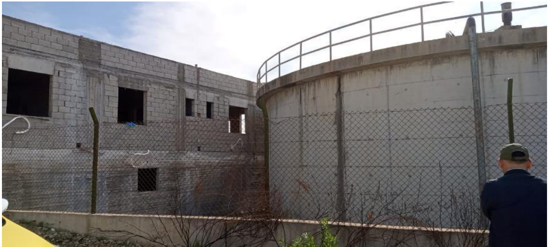
Figure 2-12: Overview of Burqin Booster Pumping Station Site (Source: Consultant)
