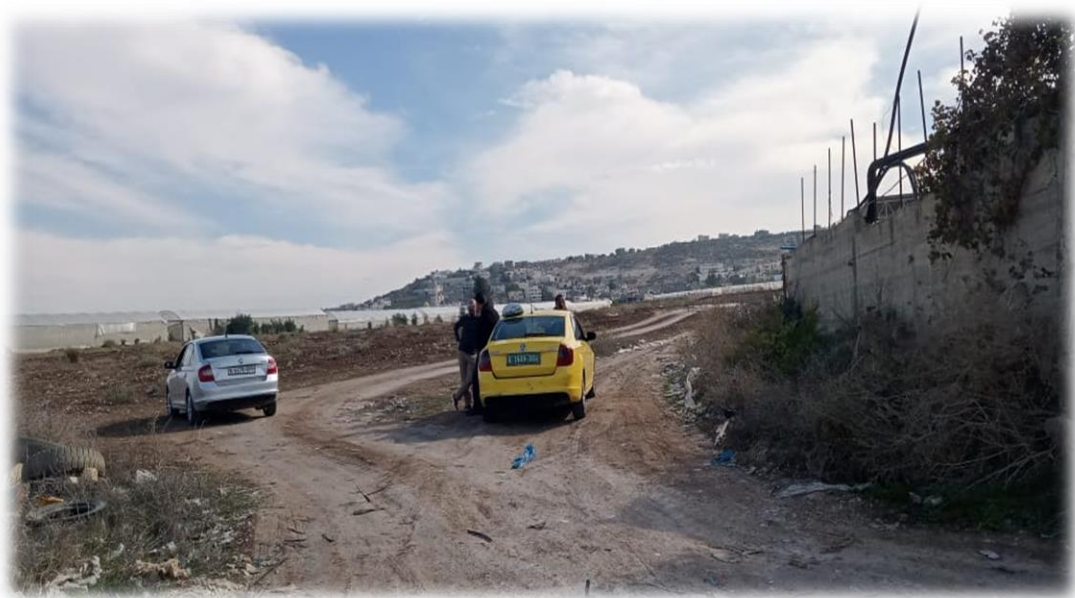
Photo for Land of Qabatiya Booster Pumping Station Adjacent to Abu Arab Well
